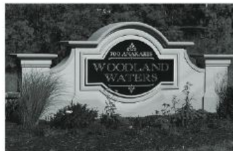
Monument Signs typically consist of a solid structural base with a framework of the same material.
