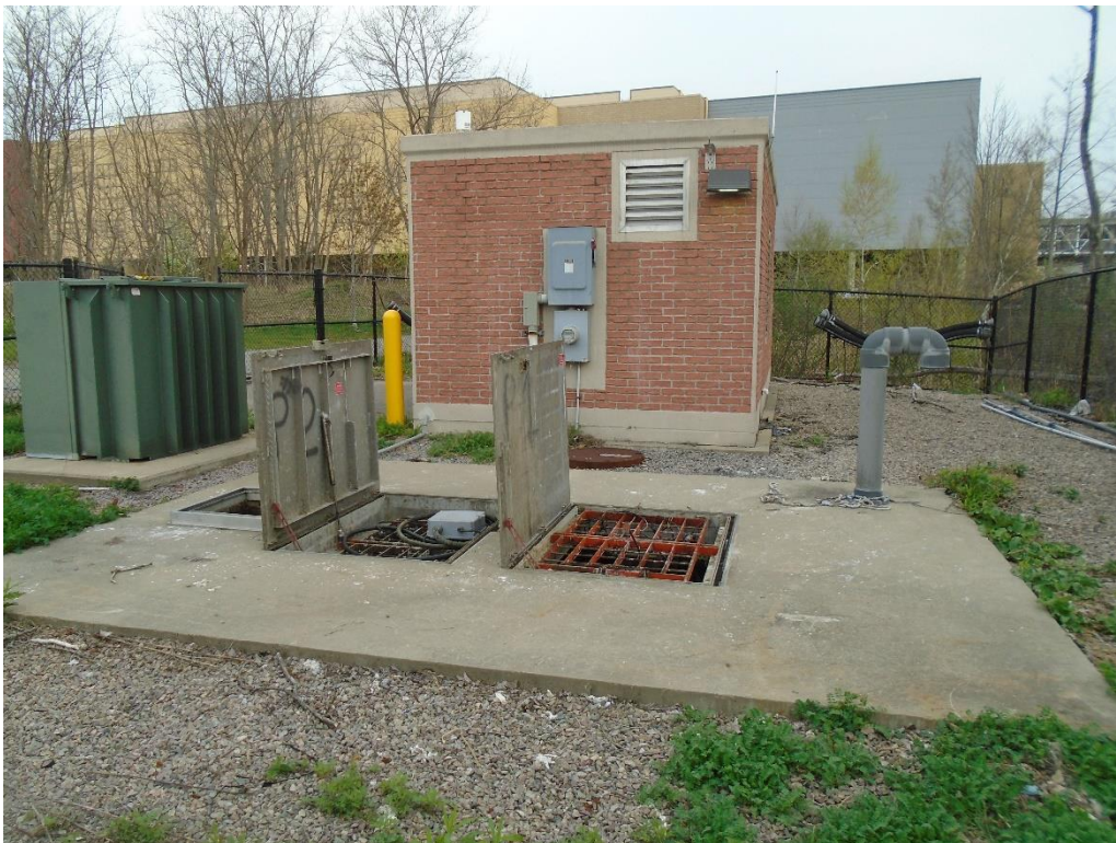
Rustcraft Road Pump Station Exterior (Side) and Wet Well/Valve Vault
