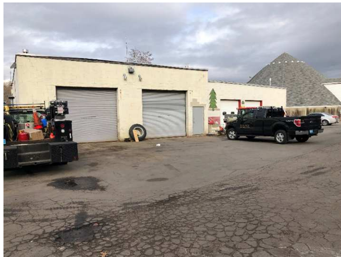
DPW Maintenance garage.
