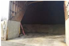
Covered salt storage
