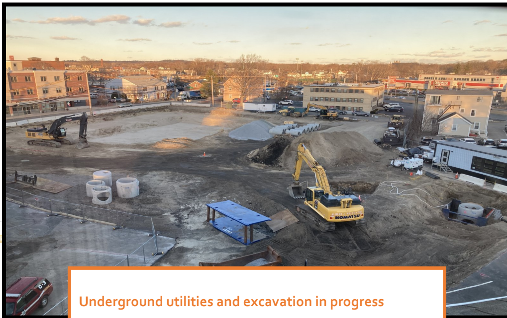
Topsoil being piled up and readied for removal
