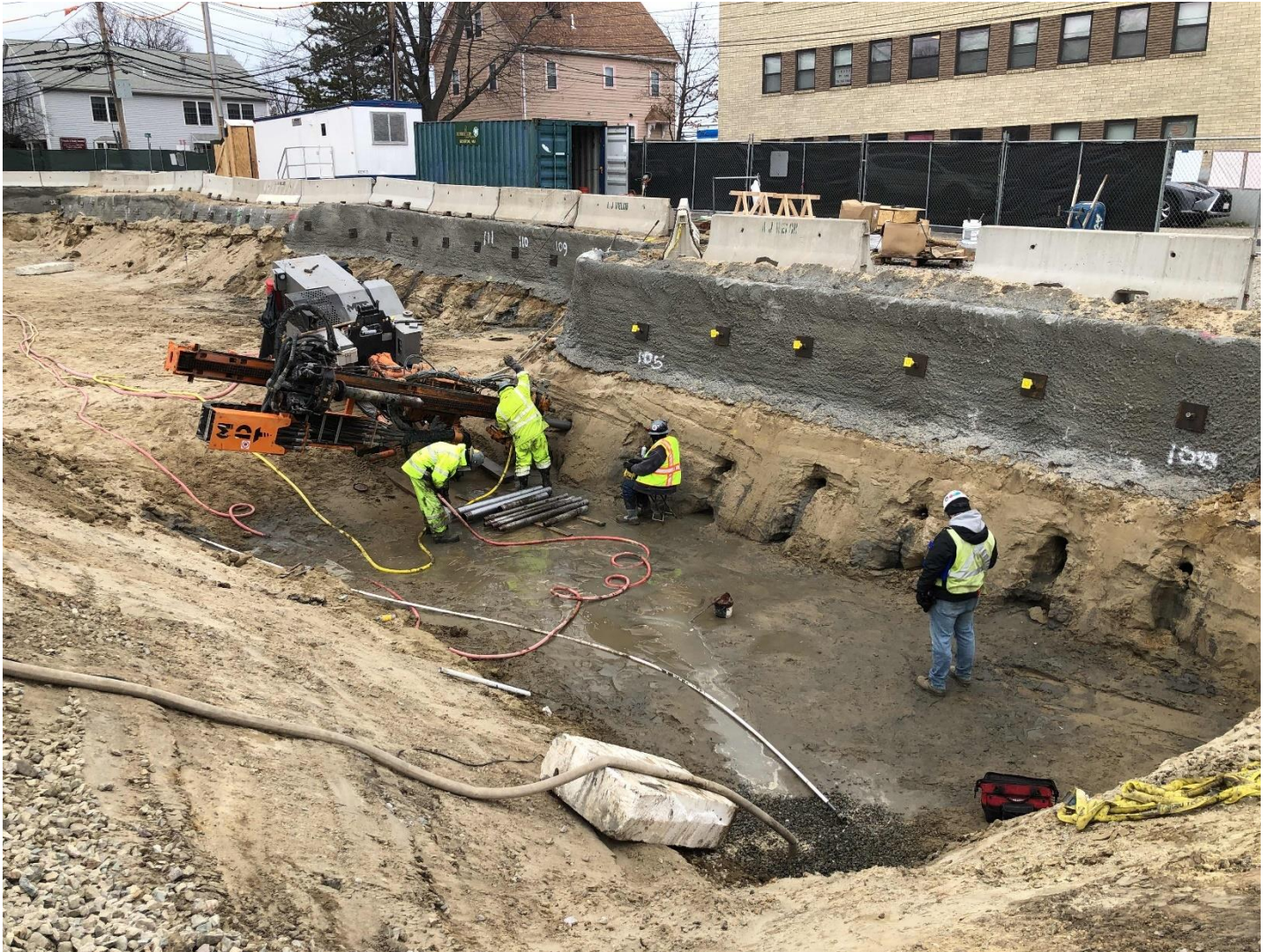
Soil nailing along Union.
