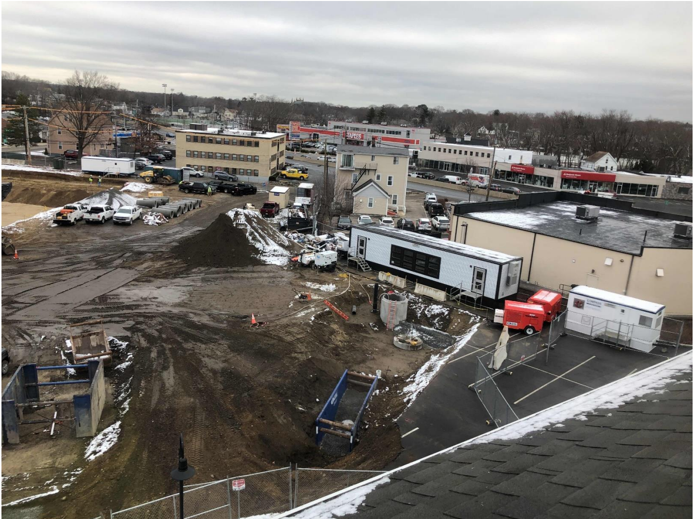
Site drainage re-routing of 36" existing to remain line is complete.
