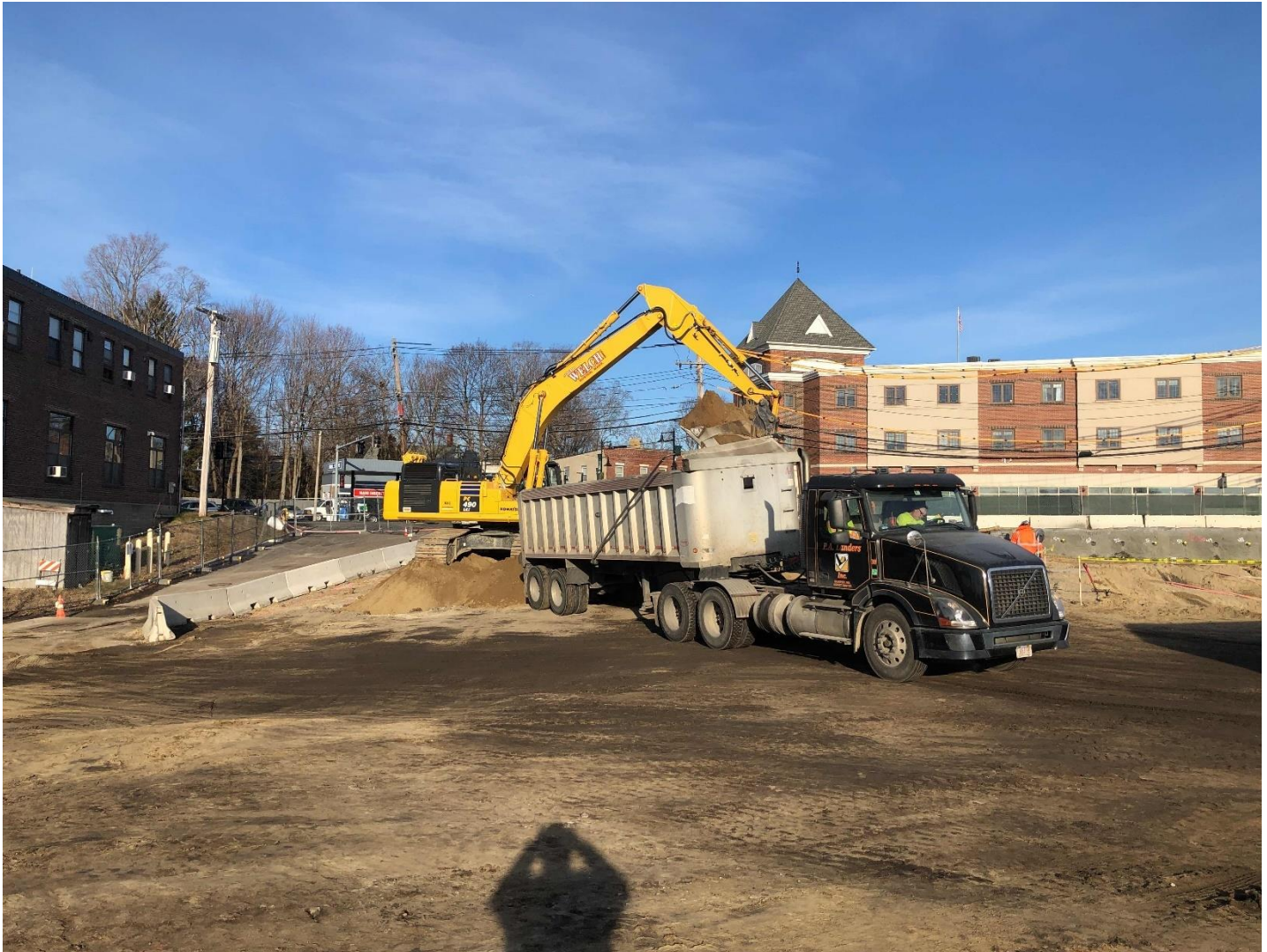
Excavation and load out continued through January
