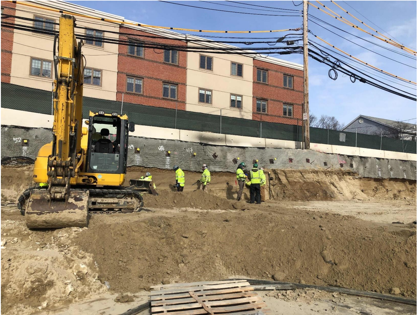
Soiling nailng, for support of excavation, along Bryant St.
