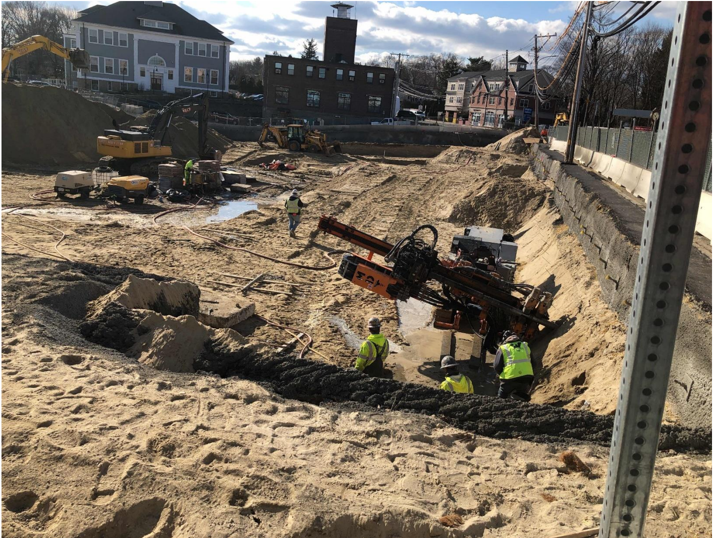
Soil nailing and site work.
