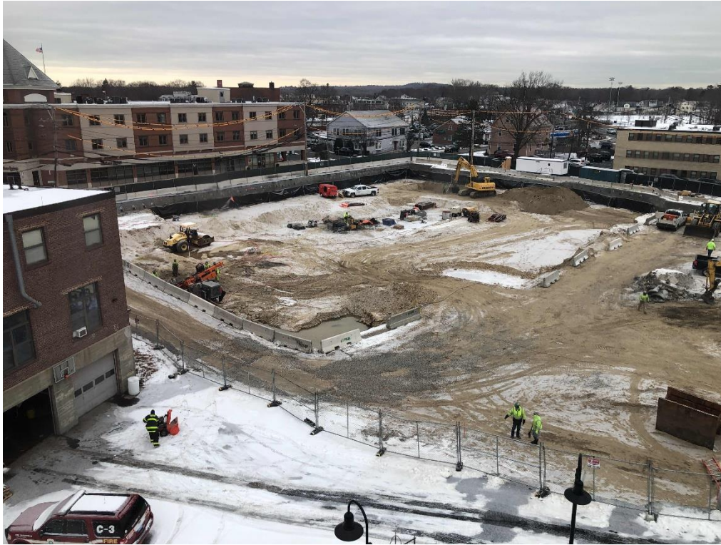
State of Support to Excavation (SOE) and excavation on 2-1-21
