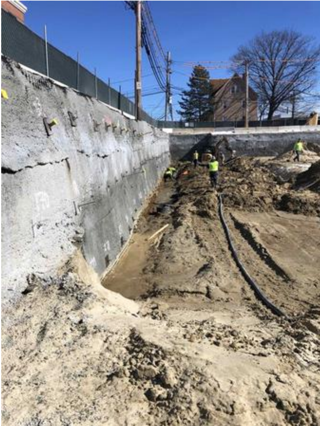
Soiling nailing, for support of excavation, along Bryant St.
