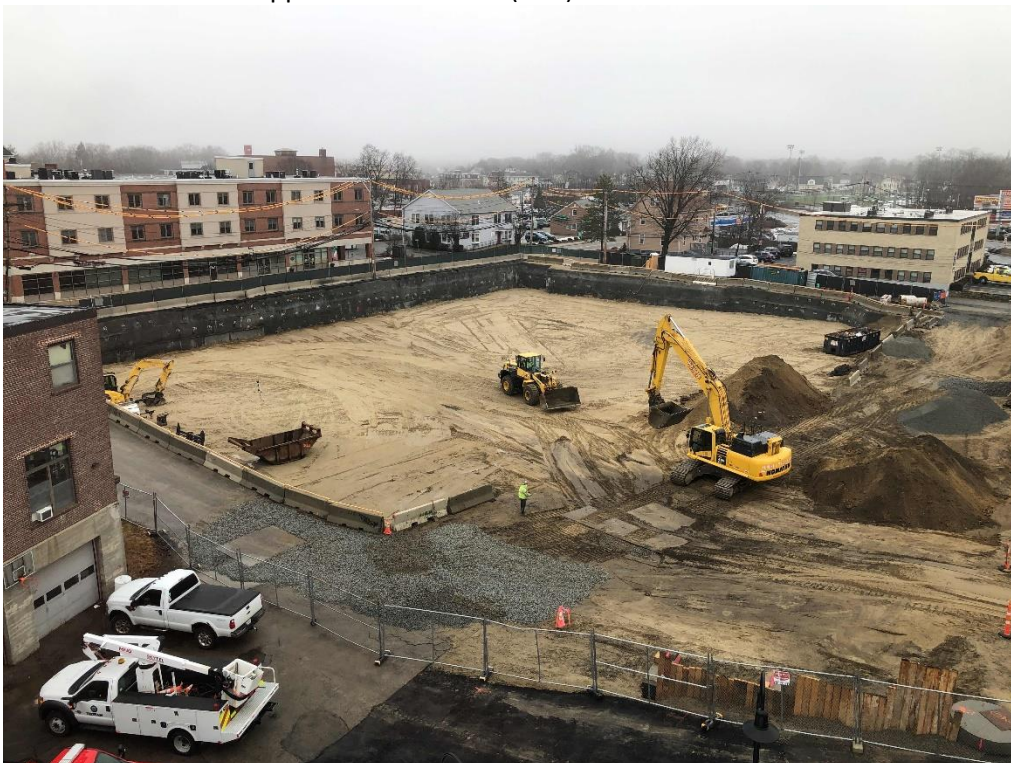
State of Support of Excavation (SOE) and excavation on 3-1-21
