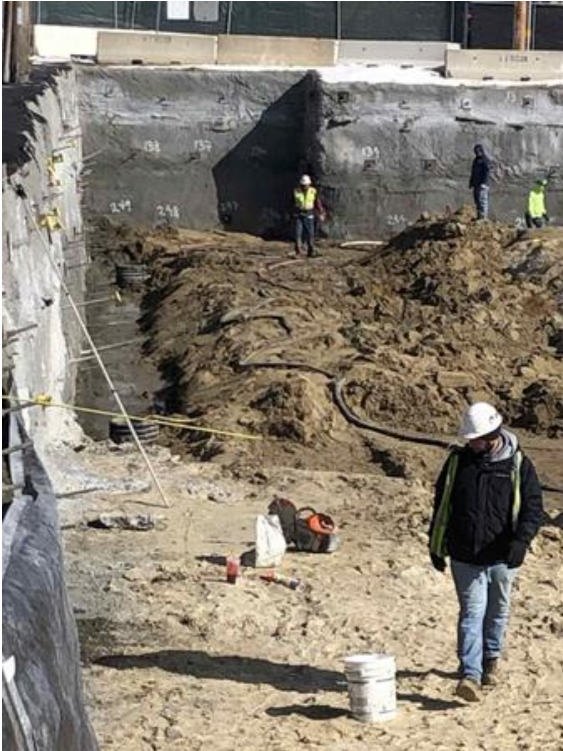
Soil nailing along existing Fire Station side
