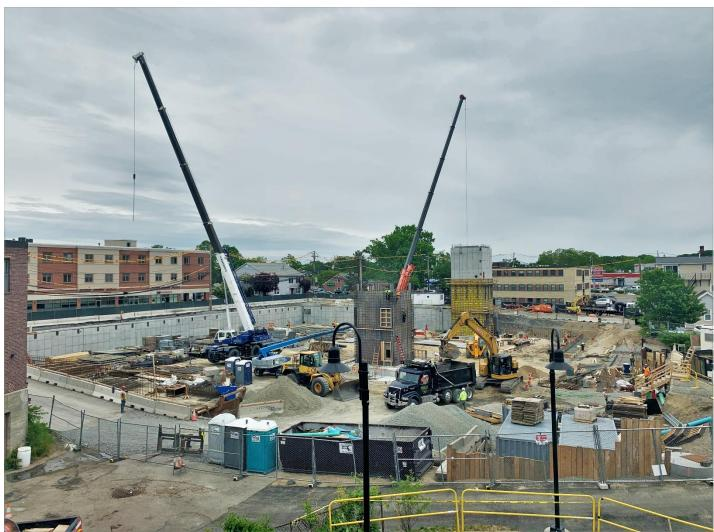
**Caption:** Photo of active construction site taken on Friday, May 28, 2021 by the Town of Dedham. Shown in the photo are stairwell #1 (center of the photo) and stairwell #2 (to the right) in progress. The shear wall framework will be removed from stairwell #2 during the week of June 1, 2021.
