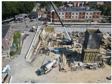
**Caption:** Aerial image of site, facing north to Bryant Street, taken on Tuesday, June 8, 2021. The shear walls for stairwell #1, shown to the right, are being formed with rebar and concrete.
