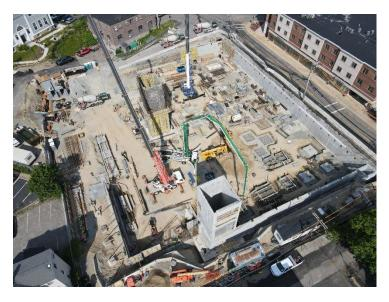
**Caption:** Aerial image of site, facing south/southwest, taken on Tuesday, June 8, 2021. The form for stairwell #2 at the bottom of the image has been removed and the shear walls have been completed.
