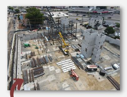
Caption (above): Aerial photo of construction site on July 21, 2021. A crane is used to raise and place each piece of steel, one a time, for installation by onsite crew members. Pieces of steel are being delivered to the site and securely stored along the west and south walls, shown at the left of this photo.
