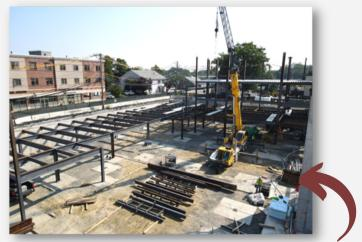
Caption (above): Aerial photo of the project site taken on July 27, 2021. The yellow crane to the right is used to raise and place each individual piece of structural steel that is secured into position.
