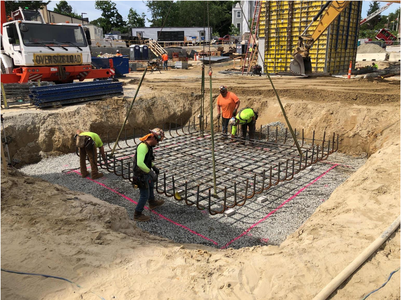
Rebar mat for footings.
