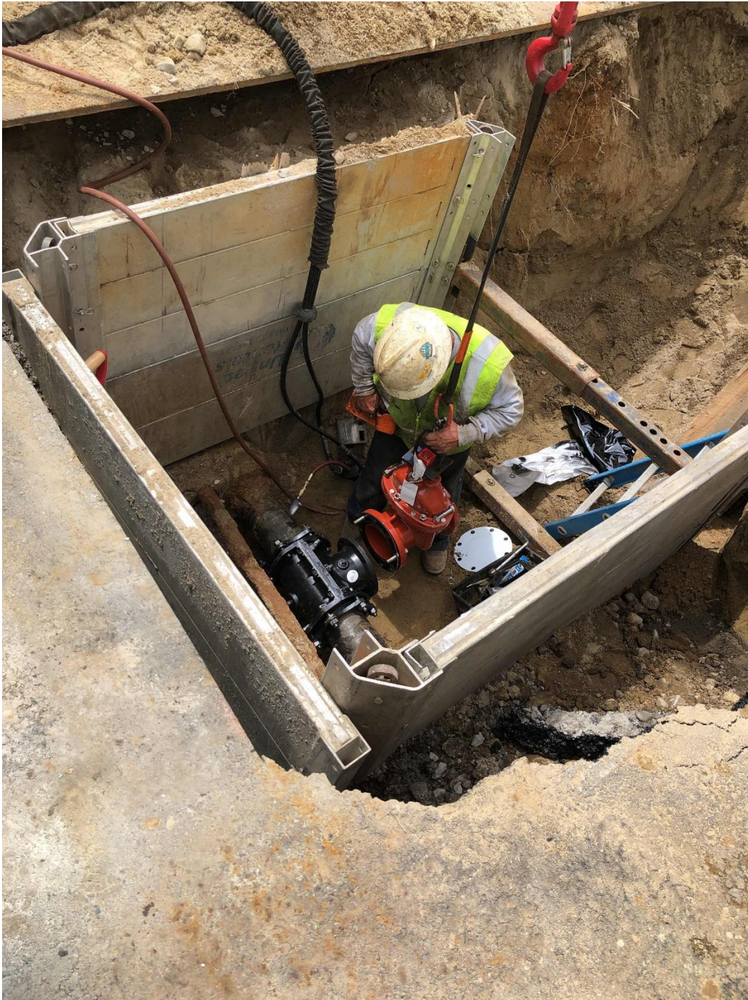
Water line tap installation
