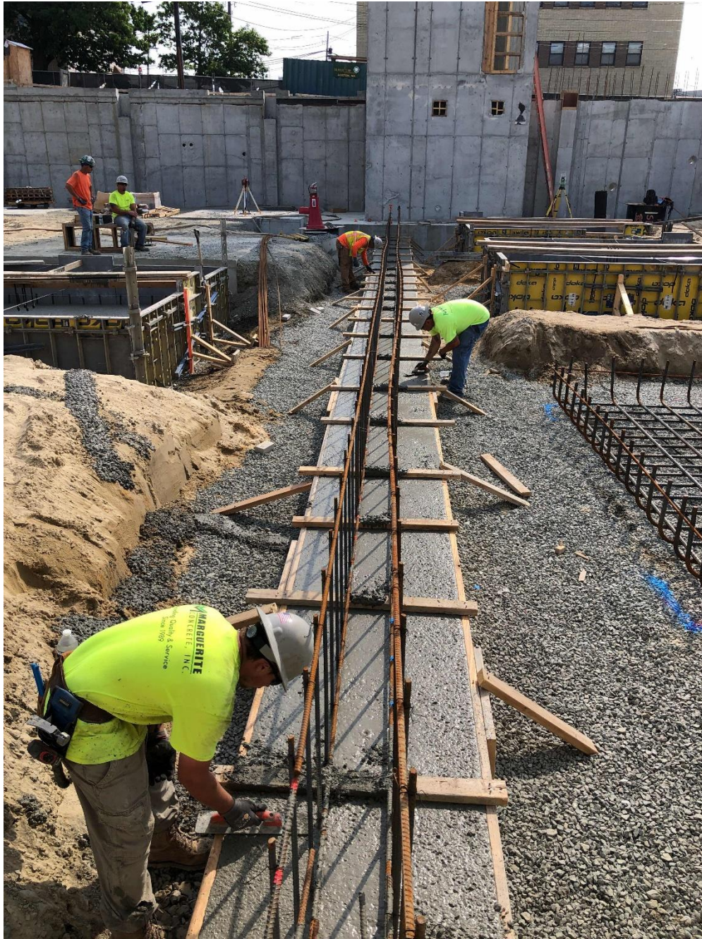
Concrete placement at interior wall footing
