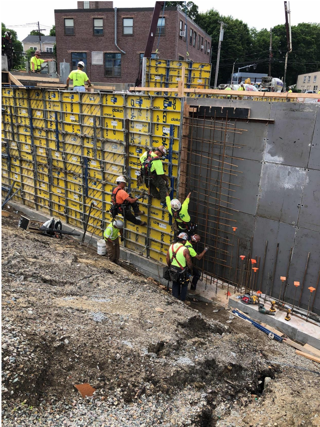
Formwork and rebar at exterior wall of parking garage.
