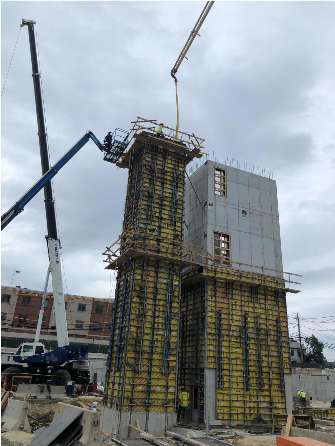
Formwork and concrete placement at elevator shaft
