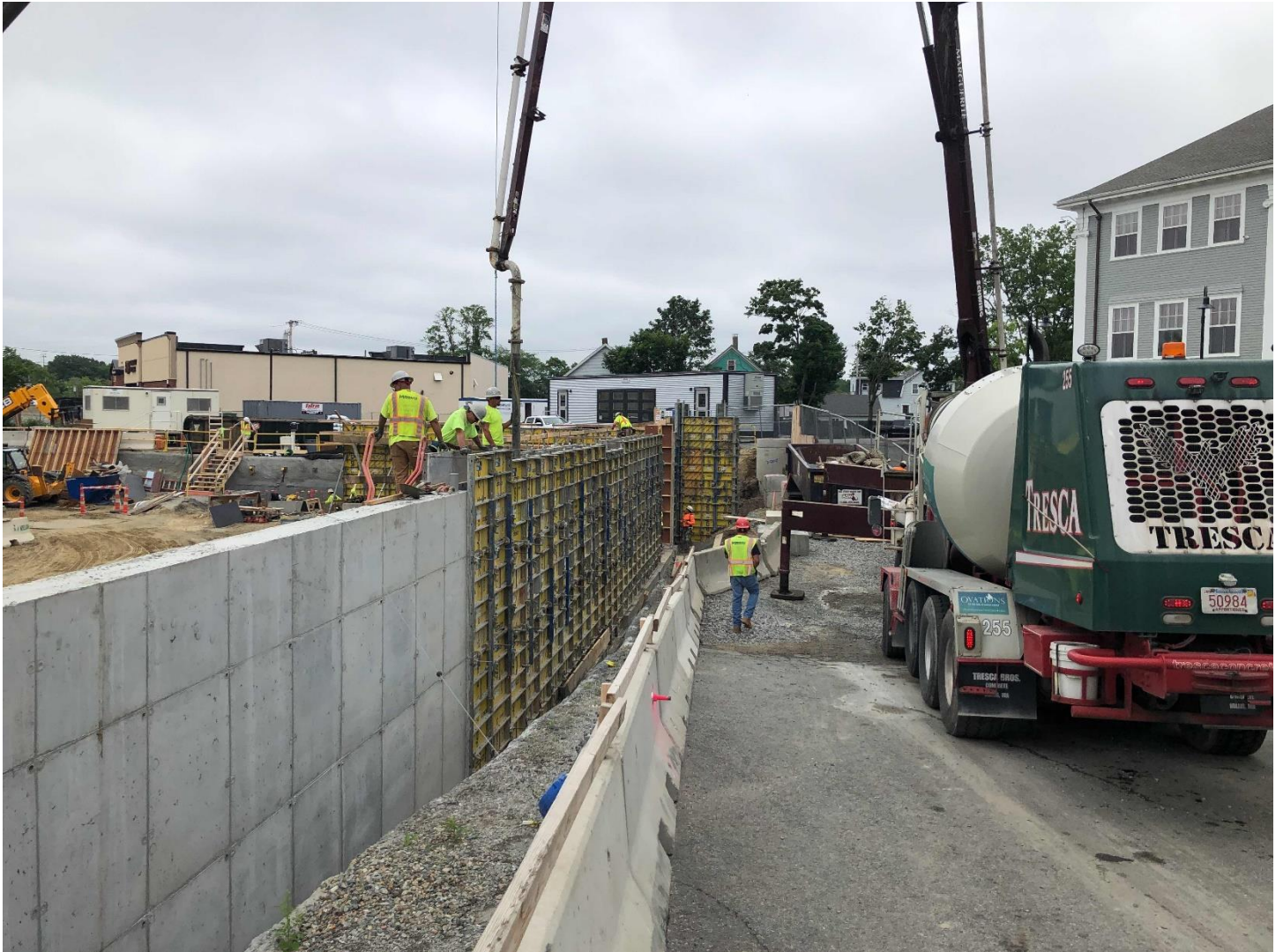
Concrete placement at exterior wall.
