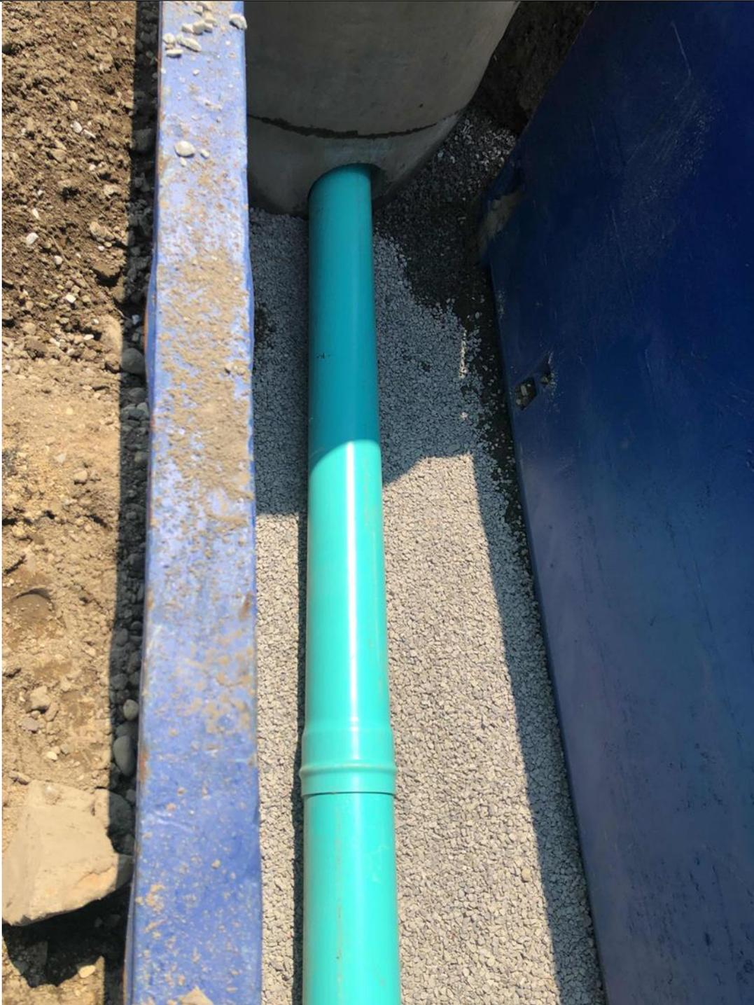
Drainage piping between Water Quality Structure #101 & new 6' diameter Drainage Manhole #208.
