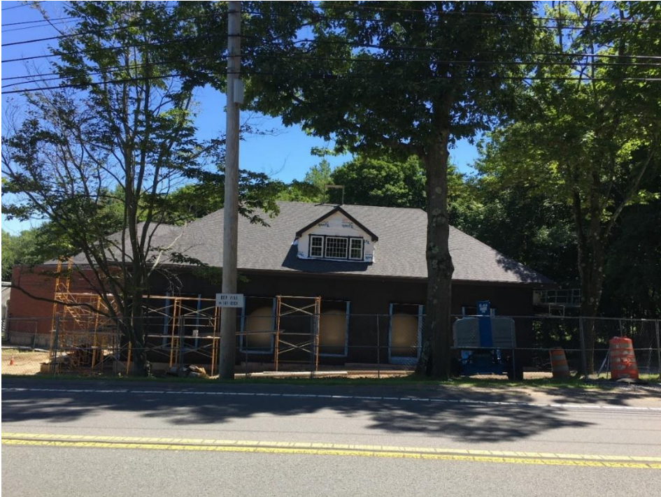
DWWD New Filter Building under construction Fall 2018
