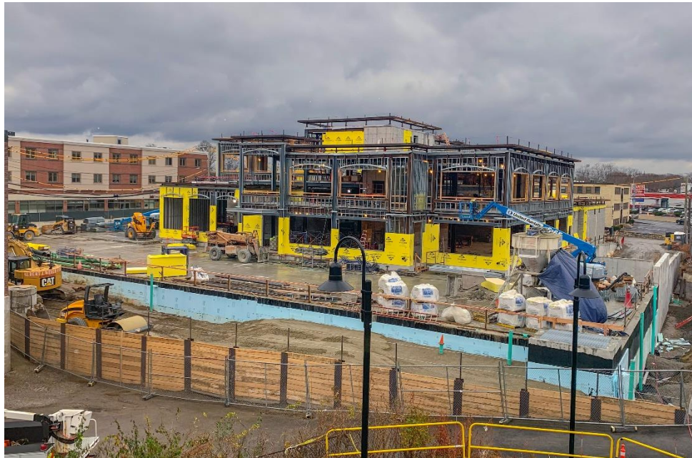
Caption: Photo of the active construction site from the north side of Town Hall on Friday, November 26, 2021. The yellow sections along the exterior walls of the building are the DensGlass sheathing, designed to resist mold and moisture.
