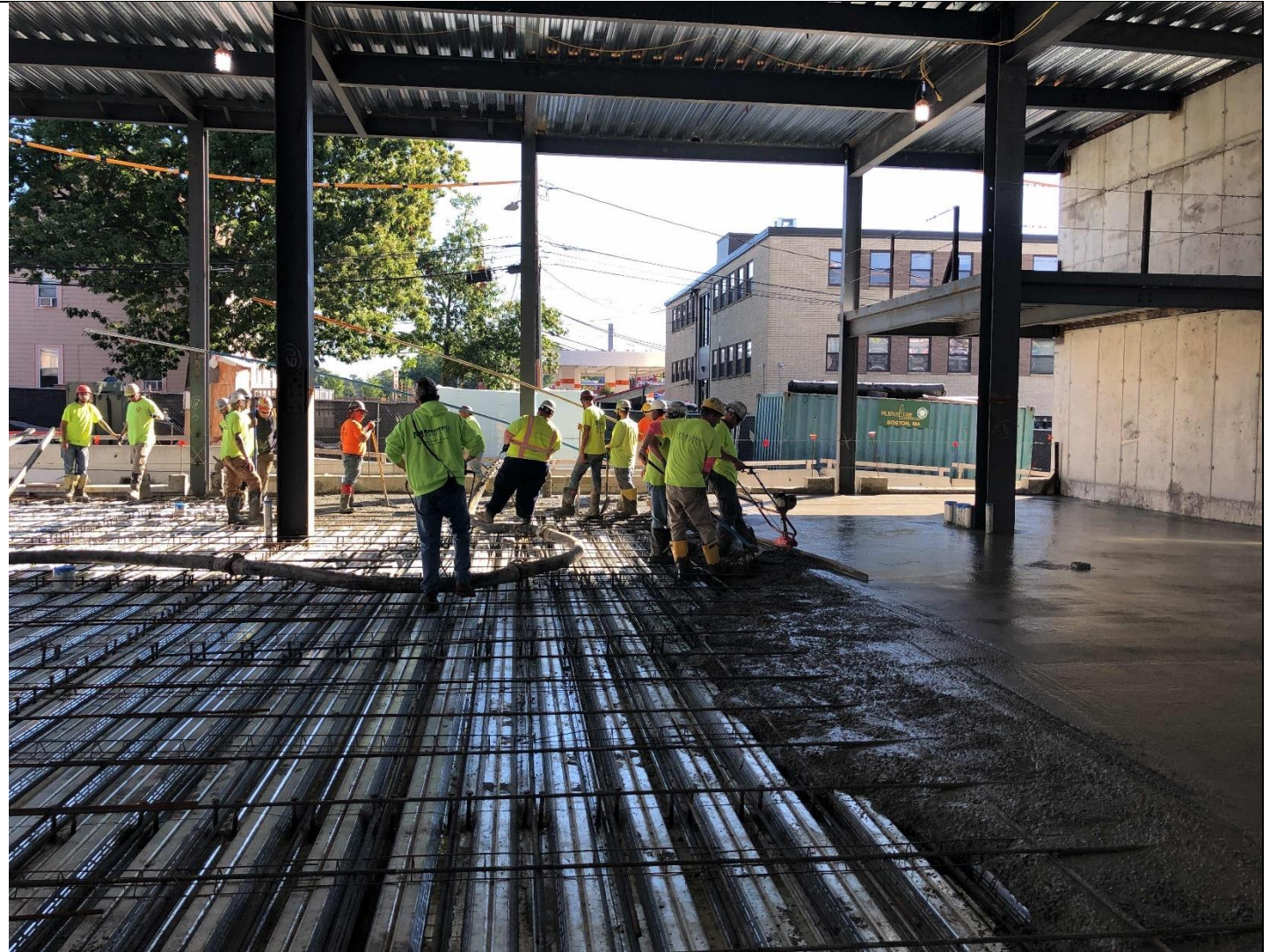
First Floor Slab-On-Deck
