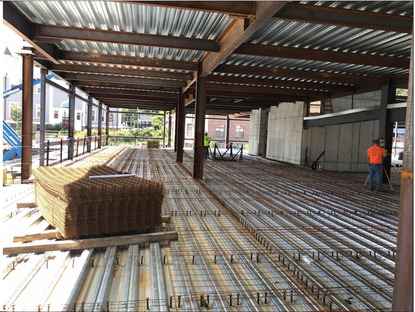
First Floor Reinforcing Steel & Mesh
