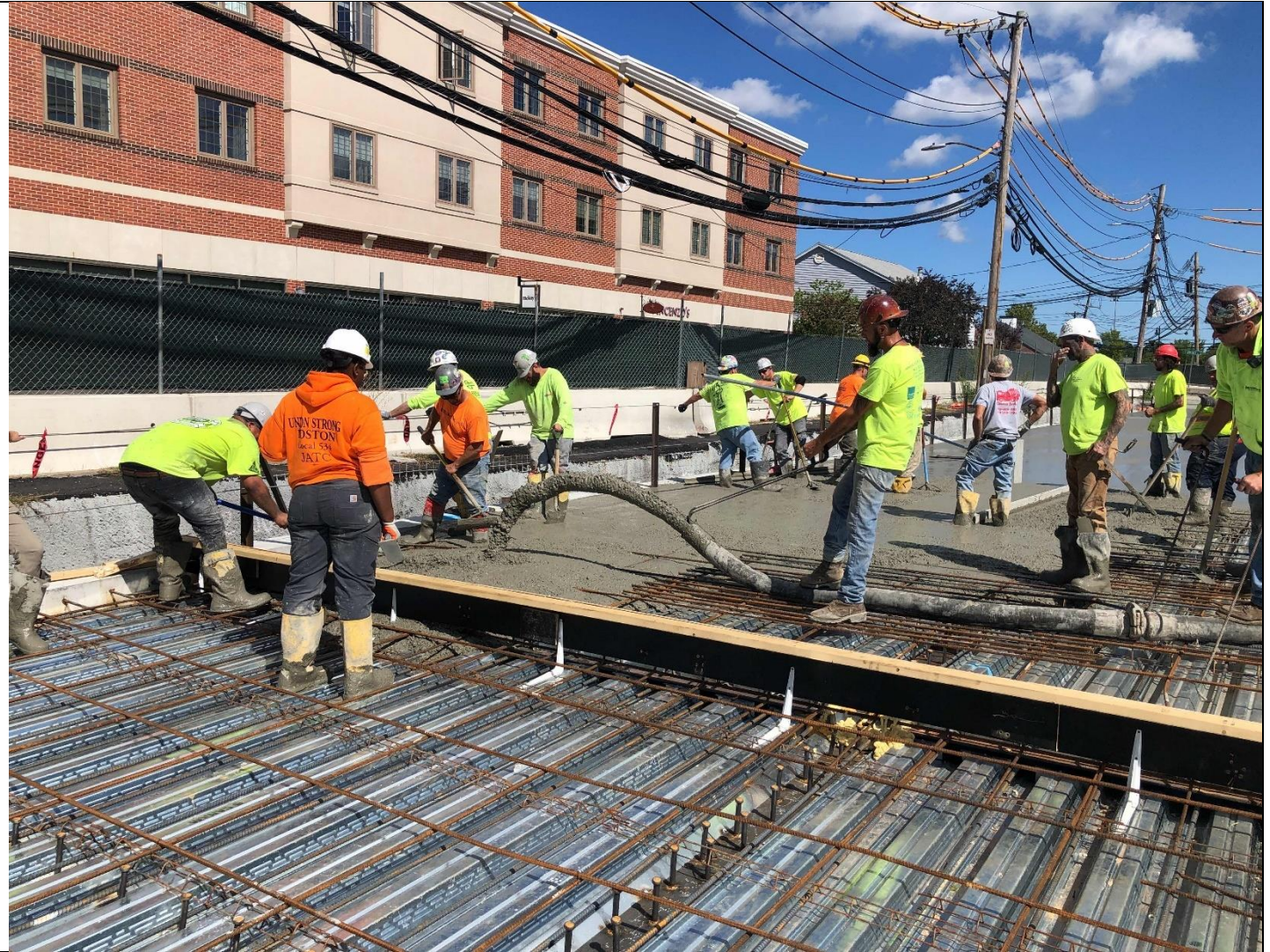
Apparatus Bay Slab-On-Deck
