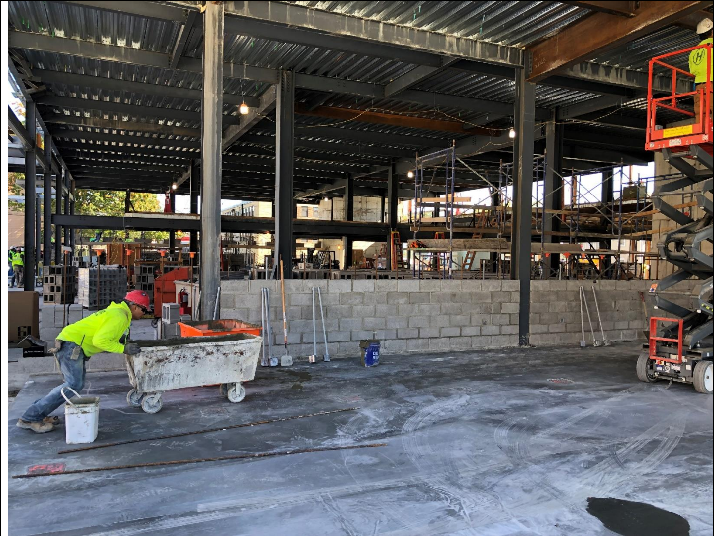
Interior Masonry CMU
