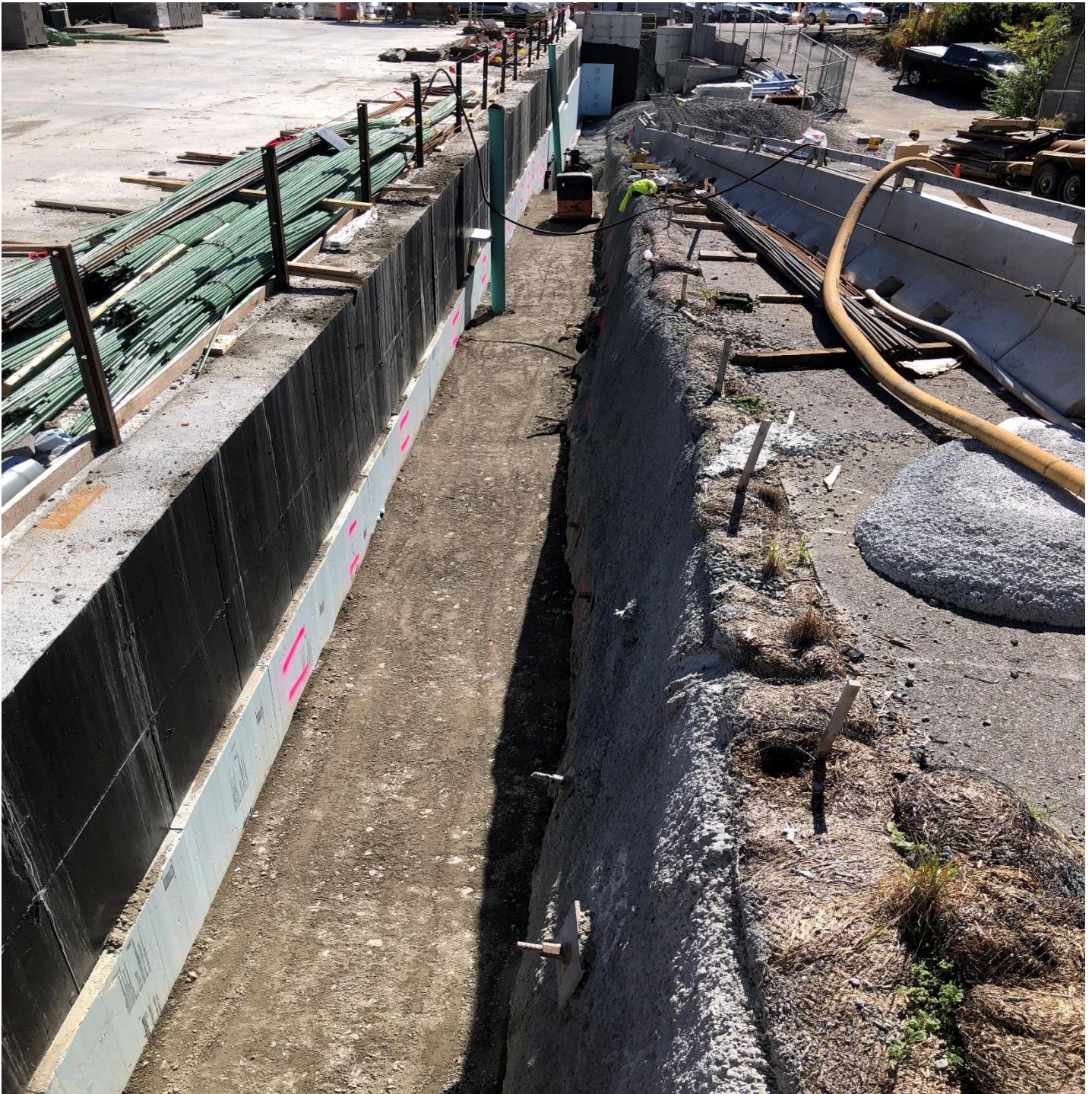
Perimeter Backfill to Grade
