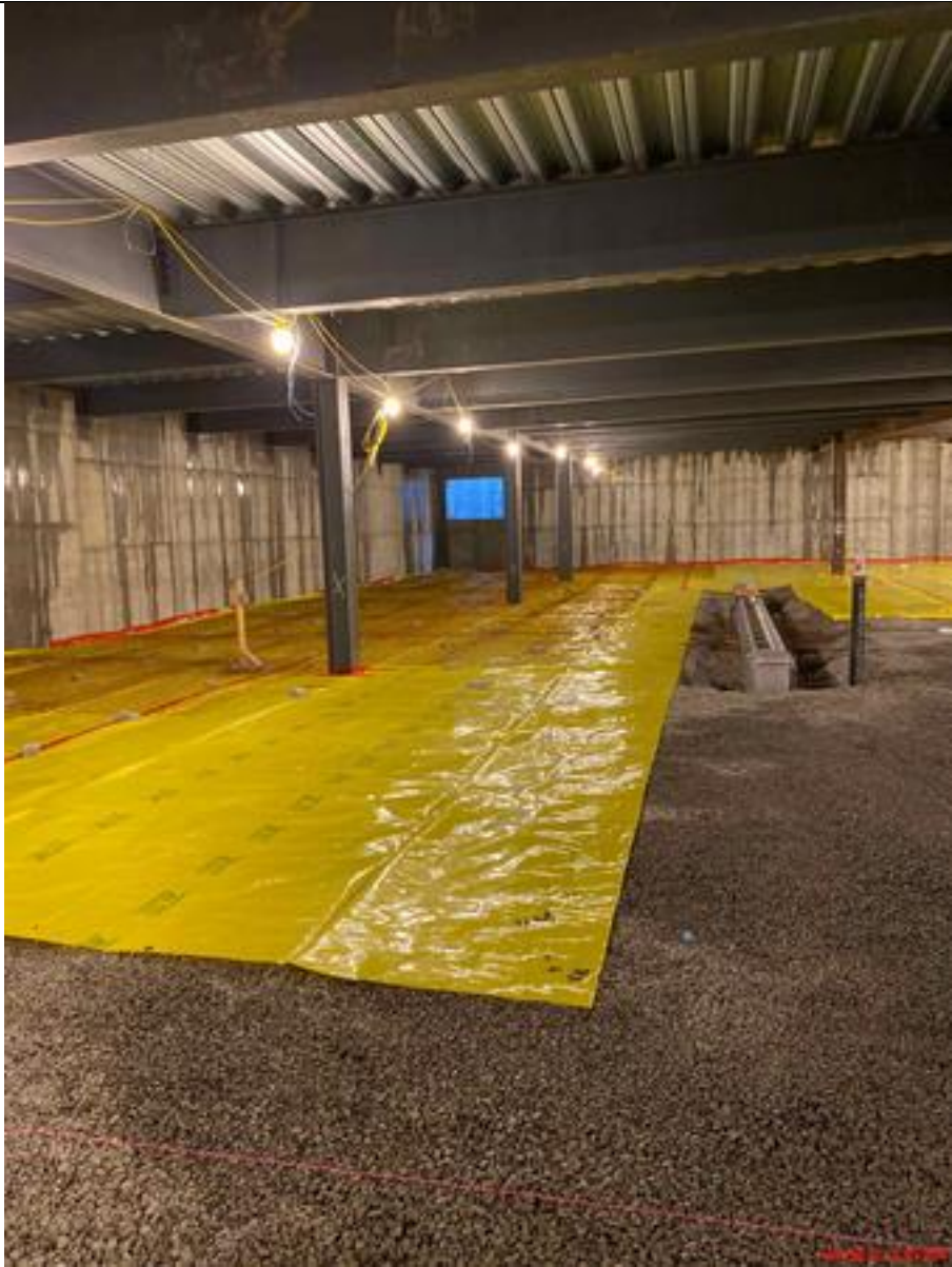
Parking Garage Stone & Stego wrap - North Half
