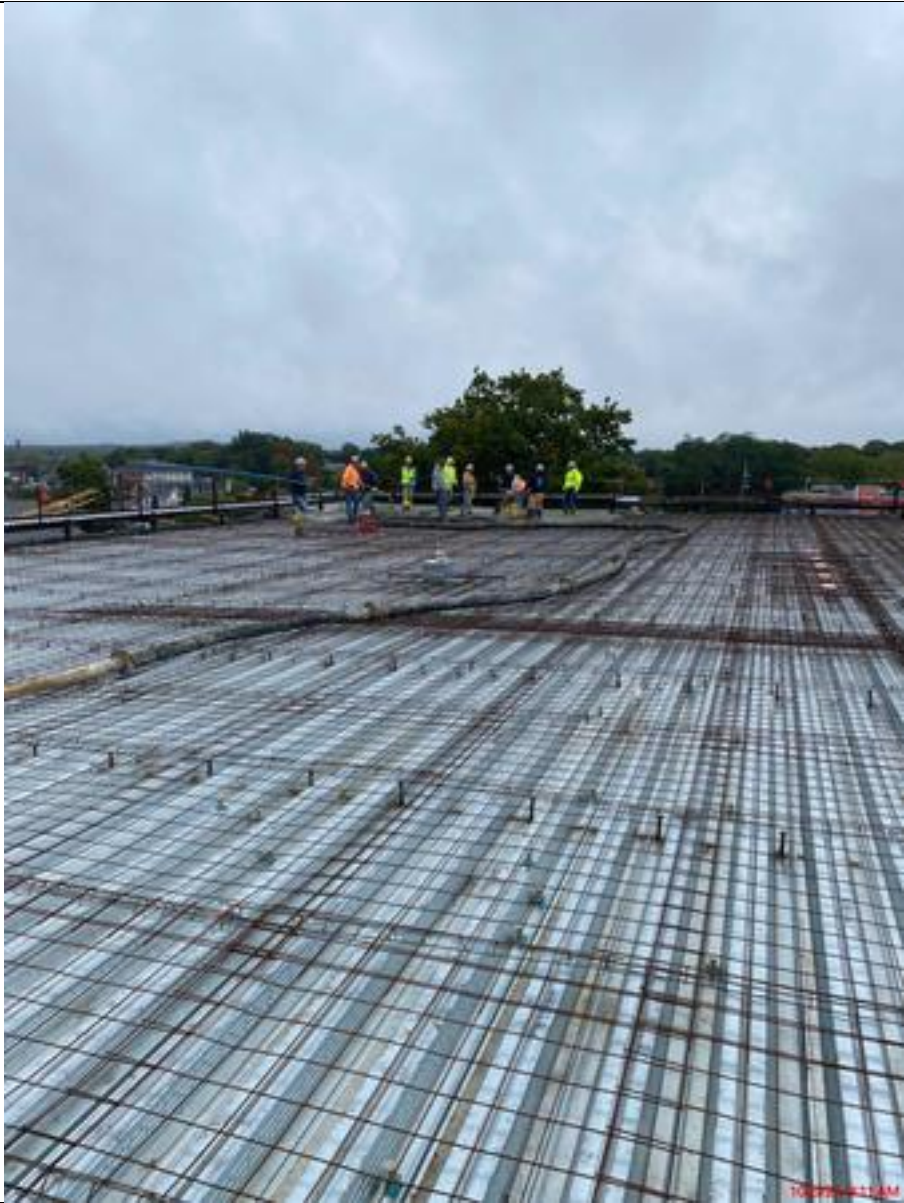
Roof Concrete/Deck Installation
