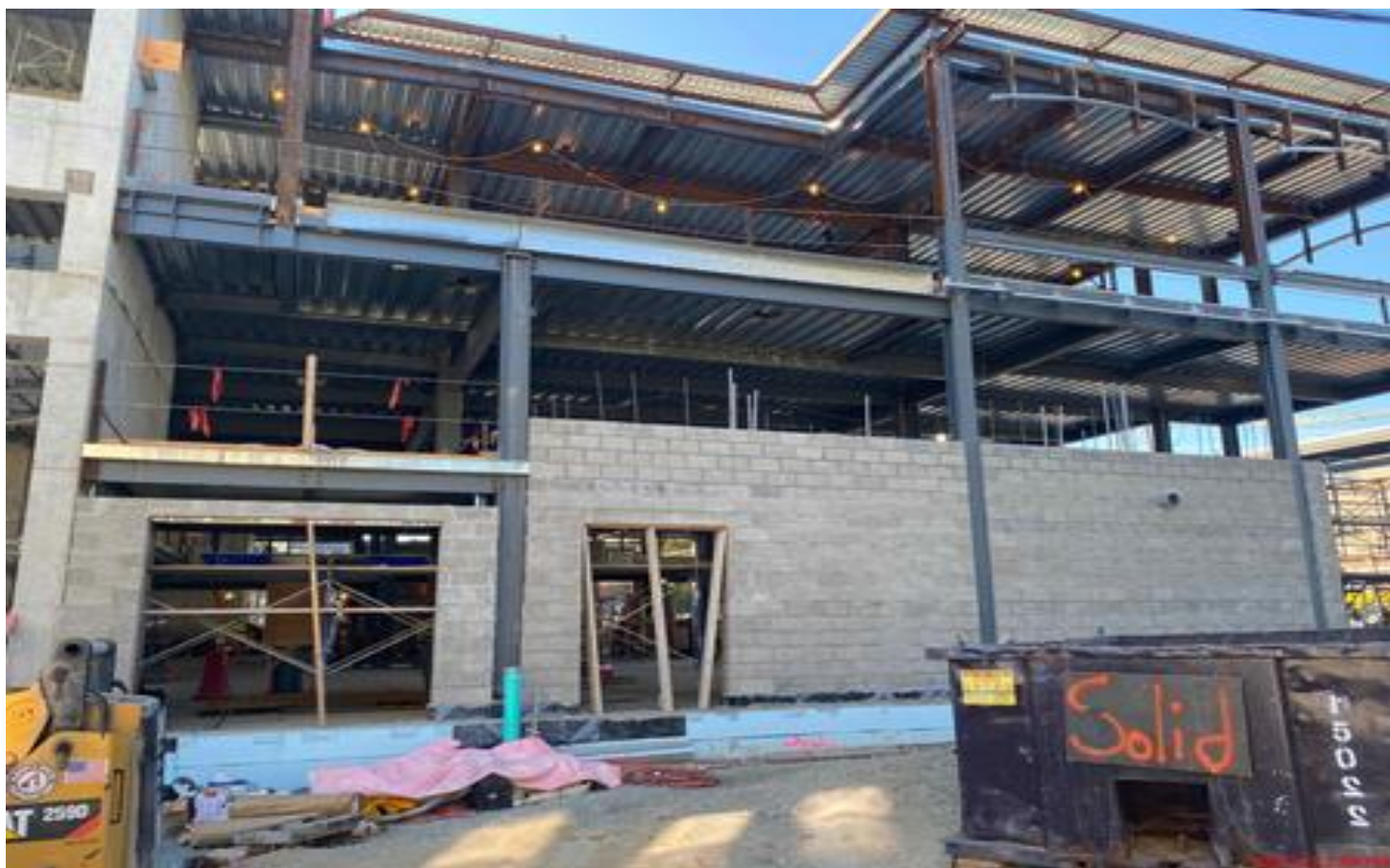
Exterior Masonry CMU
