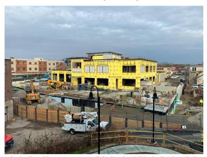
**Caption:** Photo of the active construction on Friday, December 10, 2021 taken from the north side of Town Hall. The yellow exterior of the building is the DensGlass sheathing, designed to resist moisture and mold. Crews are working to enclose the structure before temperatures drop and more snow arrives.
