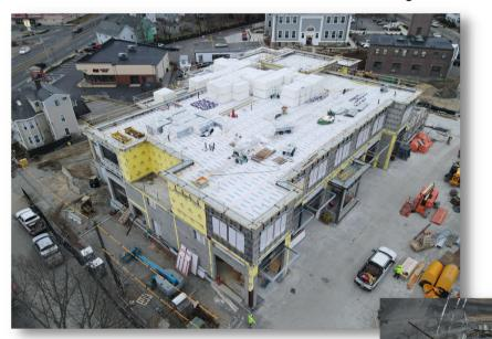
**Caption:** Photo of the active construction taken via drone on January 5, 2022 to show roofing and parapet wall materials stacked on the roof awaiting installation.
