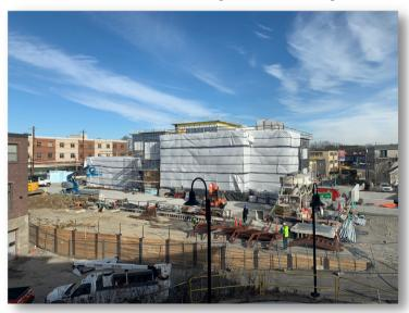
**Caption:** Photo of the active construction site taken from the north entrance to Town Hall on Friday, January 21, 2022. Sections of the metal frame stairs are lined up along the bottom of the photo in preparation for installation.
