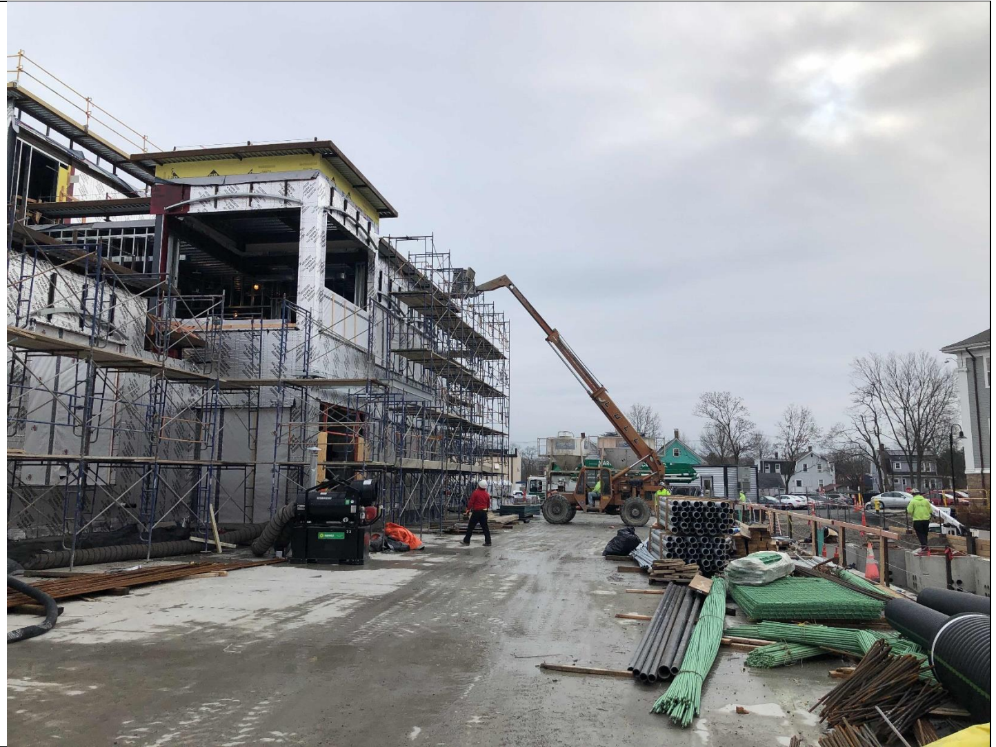
Mason Erecting Staging @ North Facade
