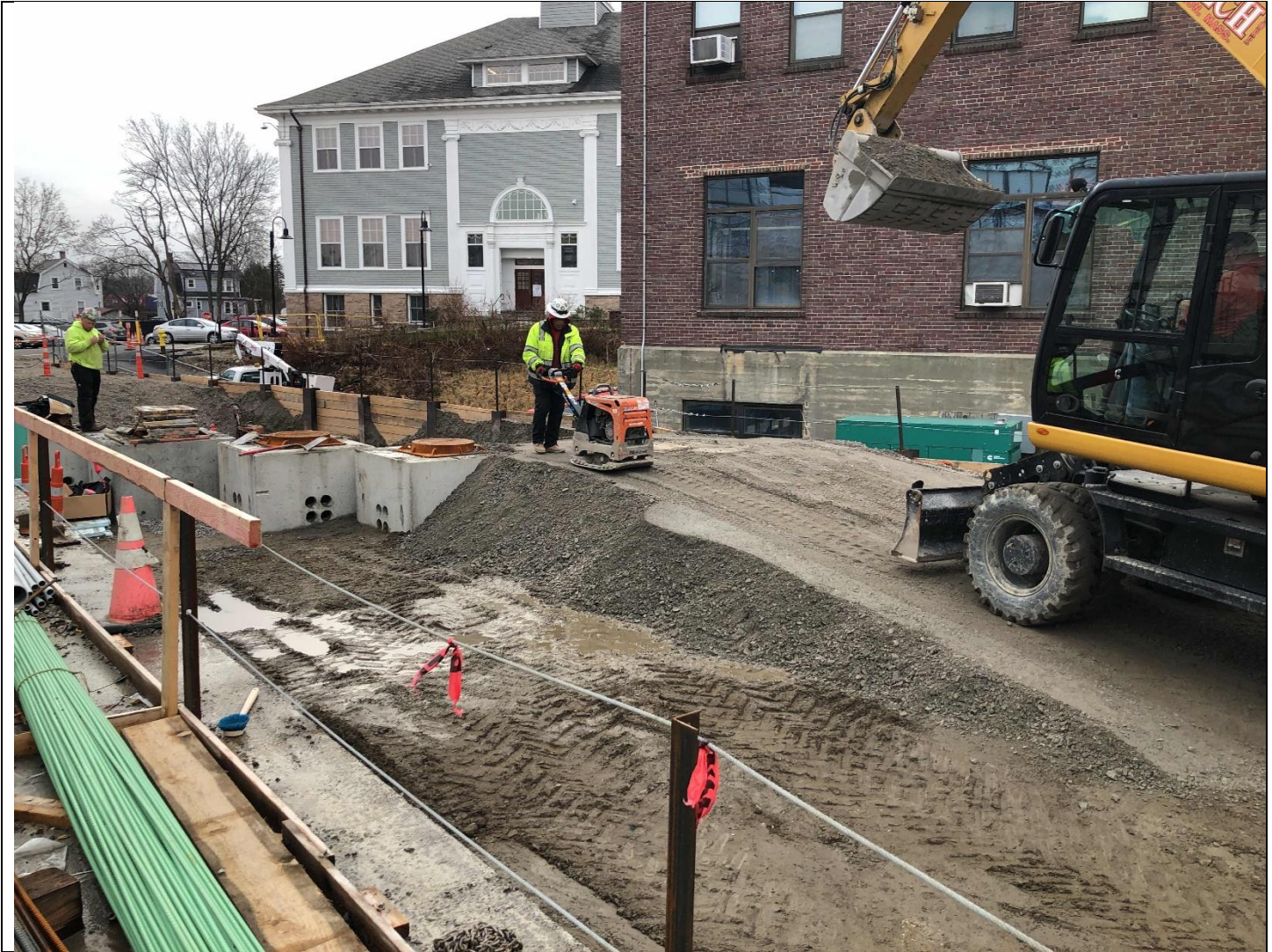
Backfilling @ ATS Duct Banks
