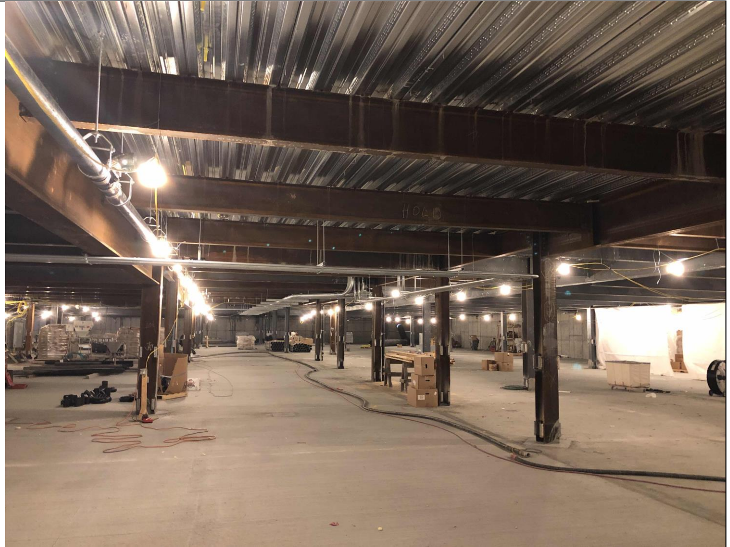
Continuing Installation MEP Utilities in Garage
