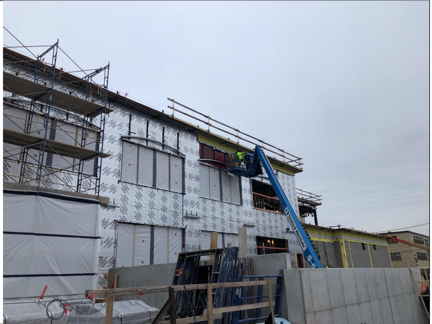
Installation of VR AIB @ Police South Facade
