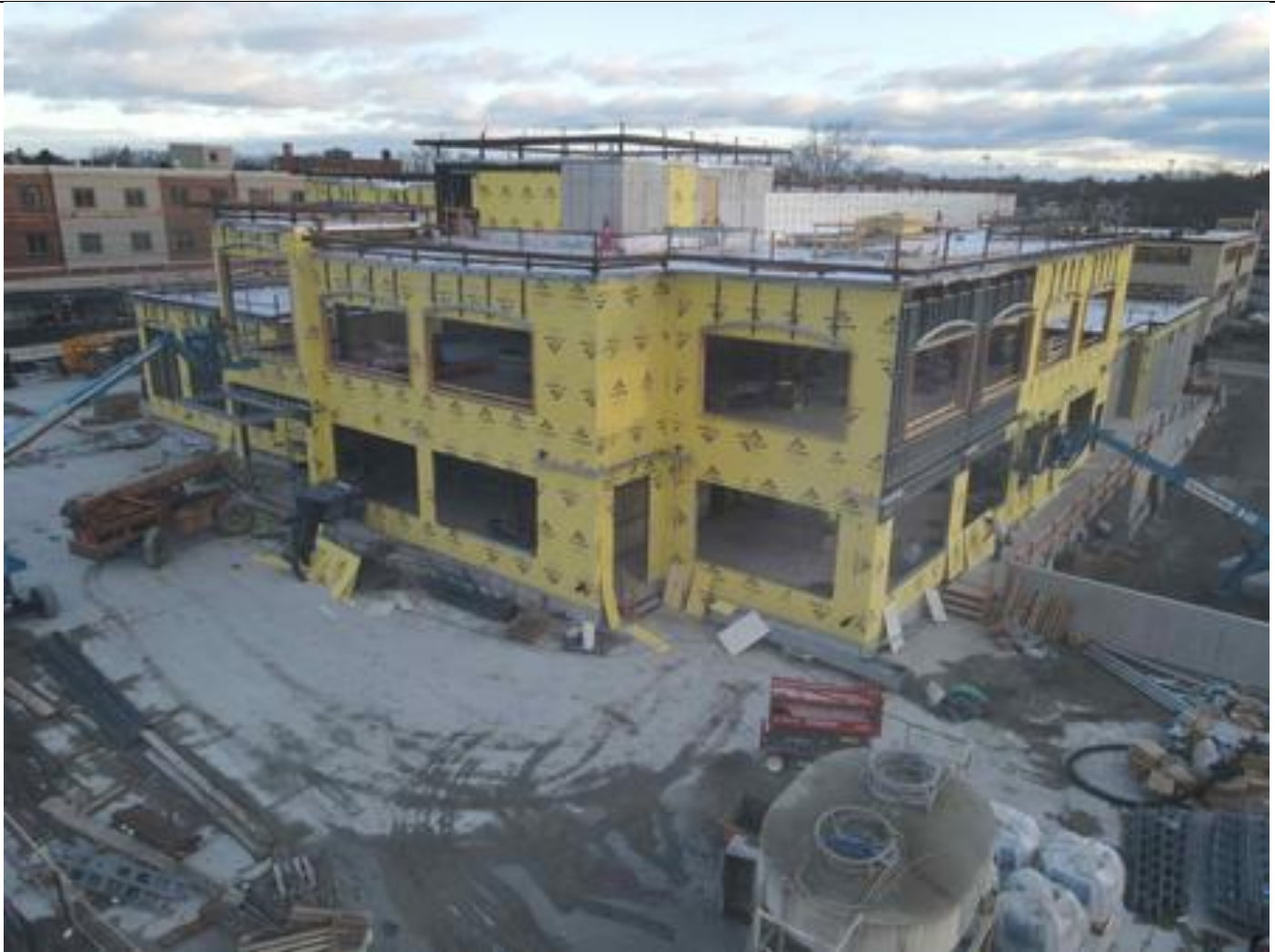
South & West Elevation Exterior Sheathing
