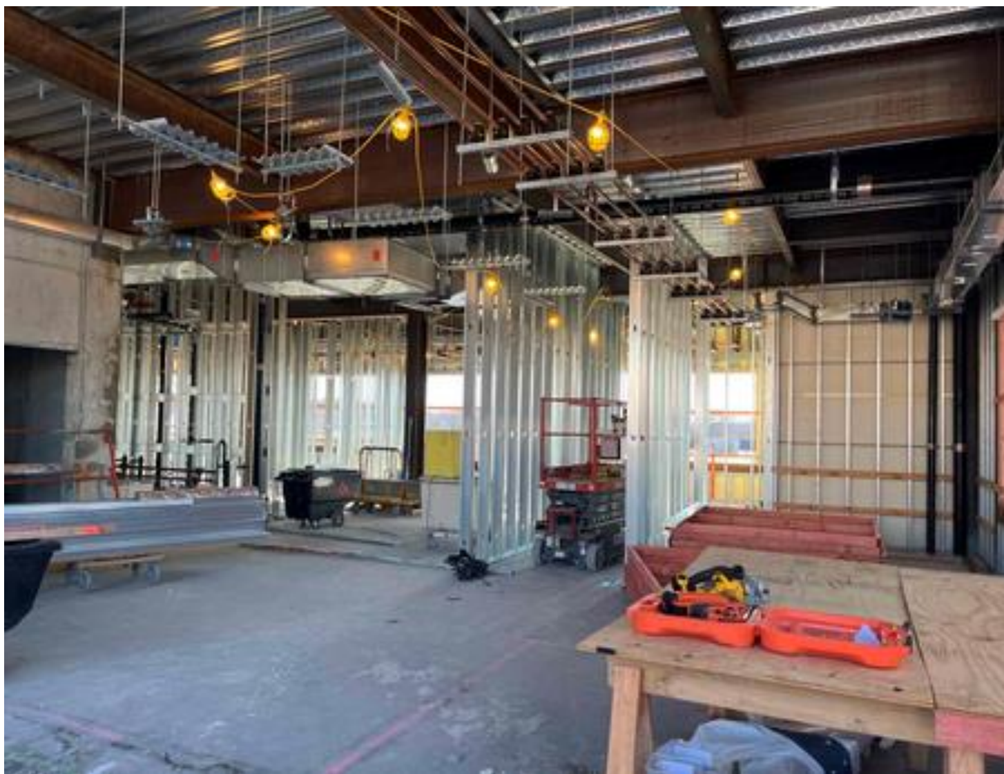
Interior Cold Formed Metal Framing
