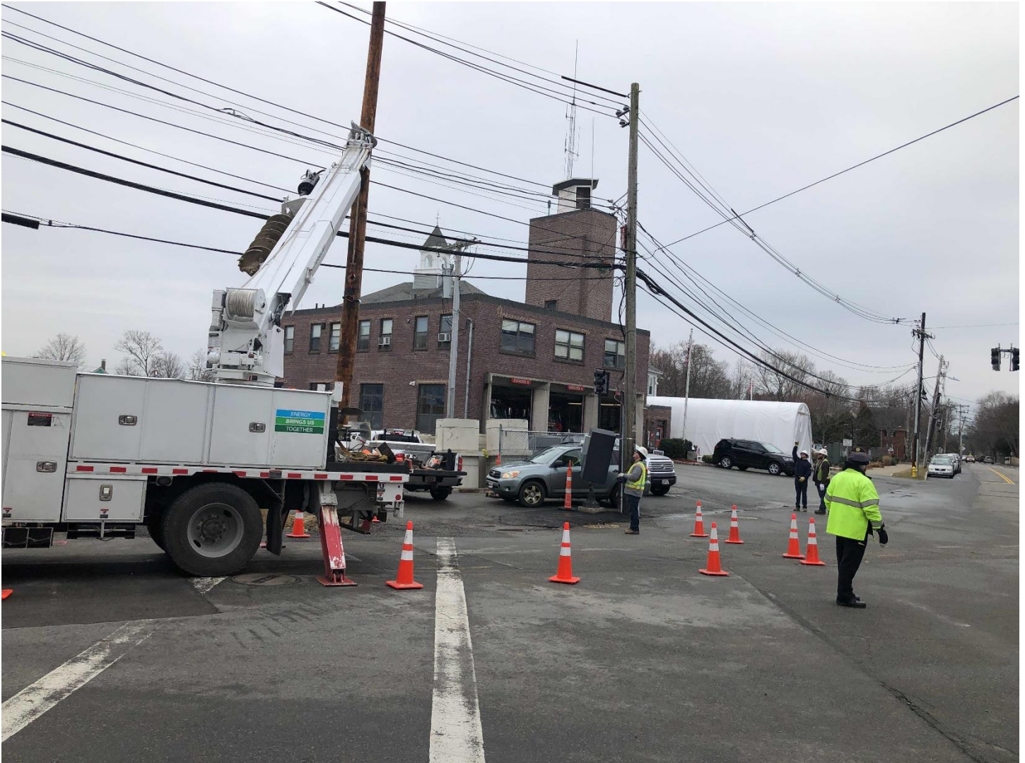
Eversource Installation of New Utility Poles
