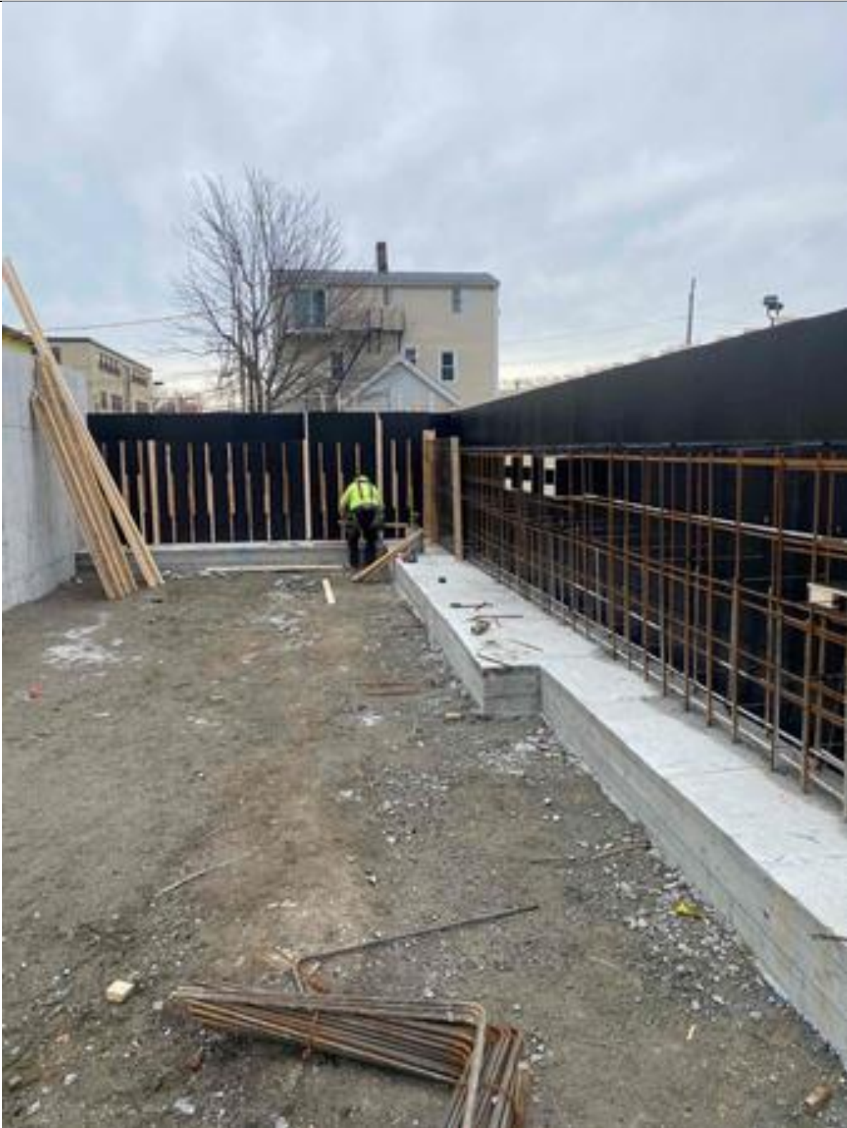
Generator Footing & Foundation Walls
