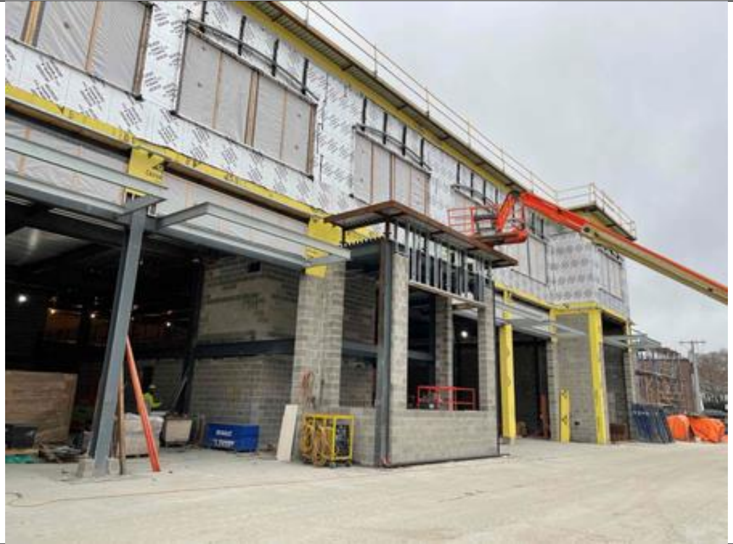
Temporary Window Installation/AVB Underway
