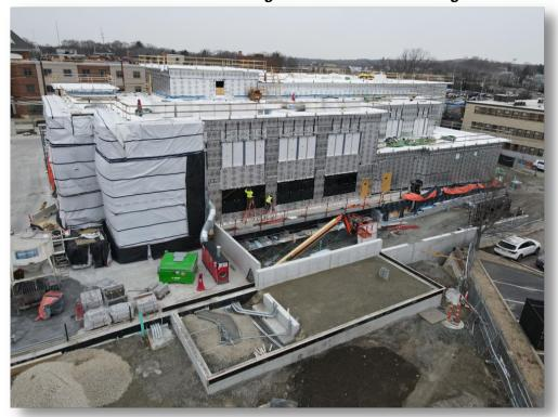
**Caption:** Photo of the active construction site, using a drone on Wednesday, March 9, 2022. Crews completed the backfill and preparations for the generator pad at the bottom of this photo. The next step is to pour the transformer pad.
