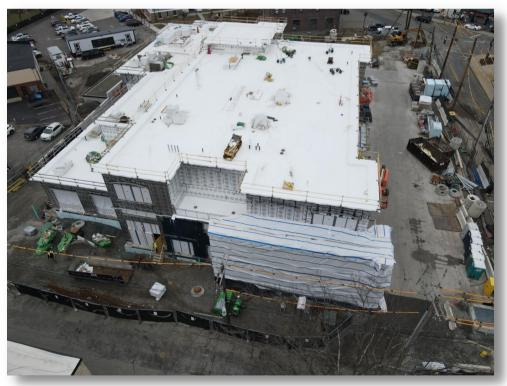
**Caption:** Photo of the active construction site, using a drone on Wednesday, March 9, 2022. Crews are still installing the exterior stone veneer, Shouldice, on the west and north sides of the building. The white plastic sheeting on the exterior of the building helps to protect the stone veneer during installation and while the mortar cures.
