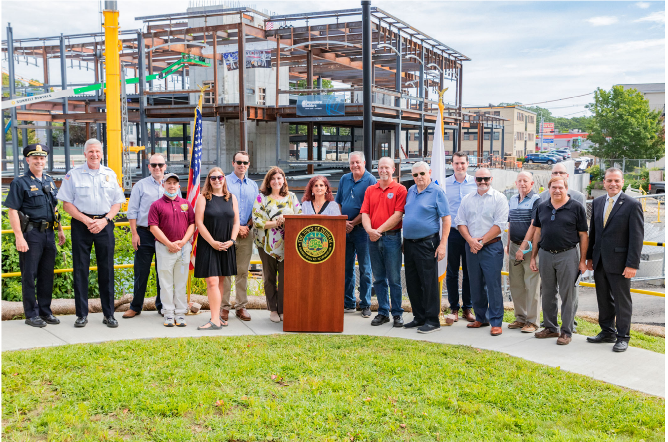
Topping off the new Public Safety facility
