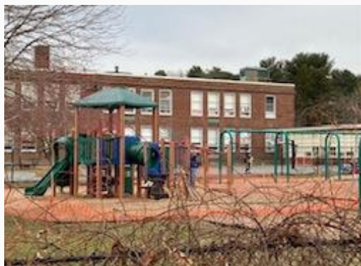
Playground before Phase 1
