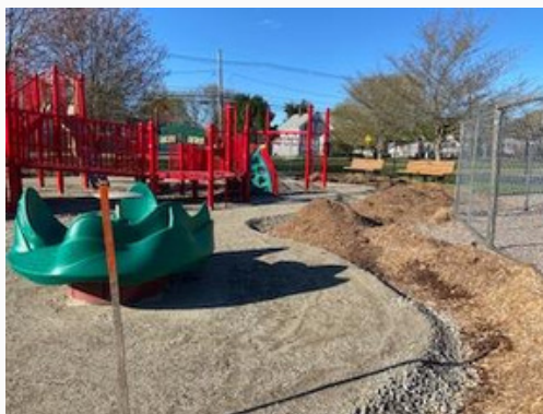
New equipment installed in Phase 1 before installation of new rubber surface
