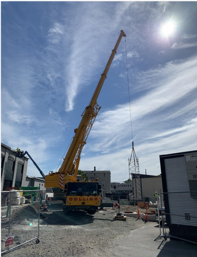
CAPTION: Photo of crane lifting section of cell tower for installation within the site boundaries of the new Public Safety Building, take on Wednesday, June 29, 2022.
