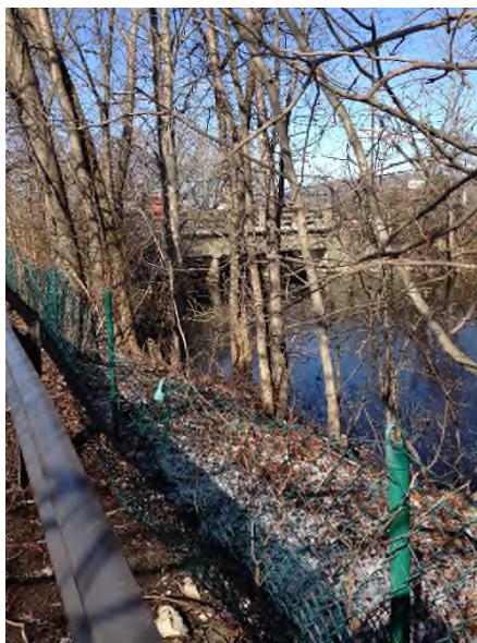
Photo 1. View upstream of Mother Brook facing Incinerator Road crossing.
