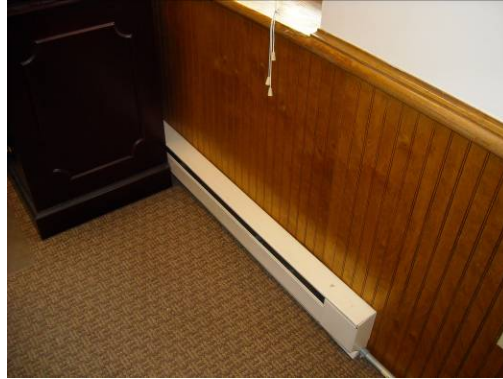
Electric Baseboard Heating
