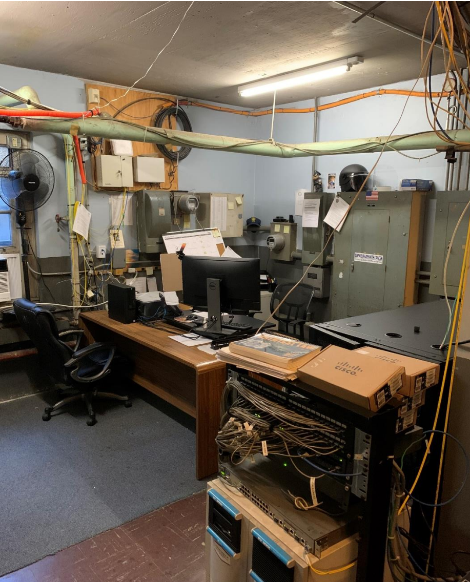
Office Located in Electrical Room
