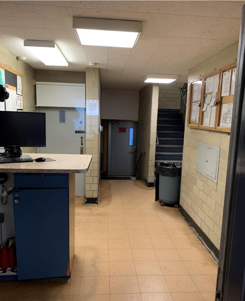
Hallway used for booking presents a significant security risk. Also used for roll call setting an unprofessional tone.
