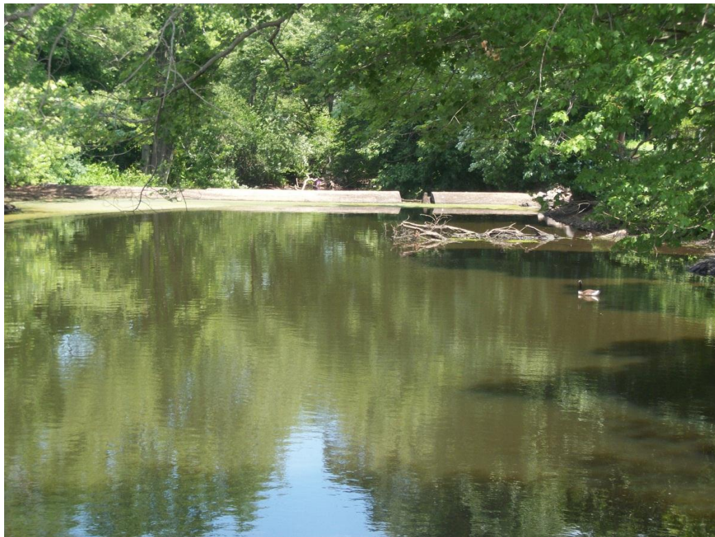
Photo 10: Upstream view of dam.
