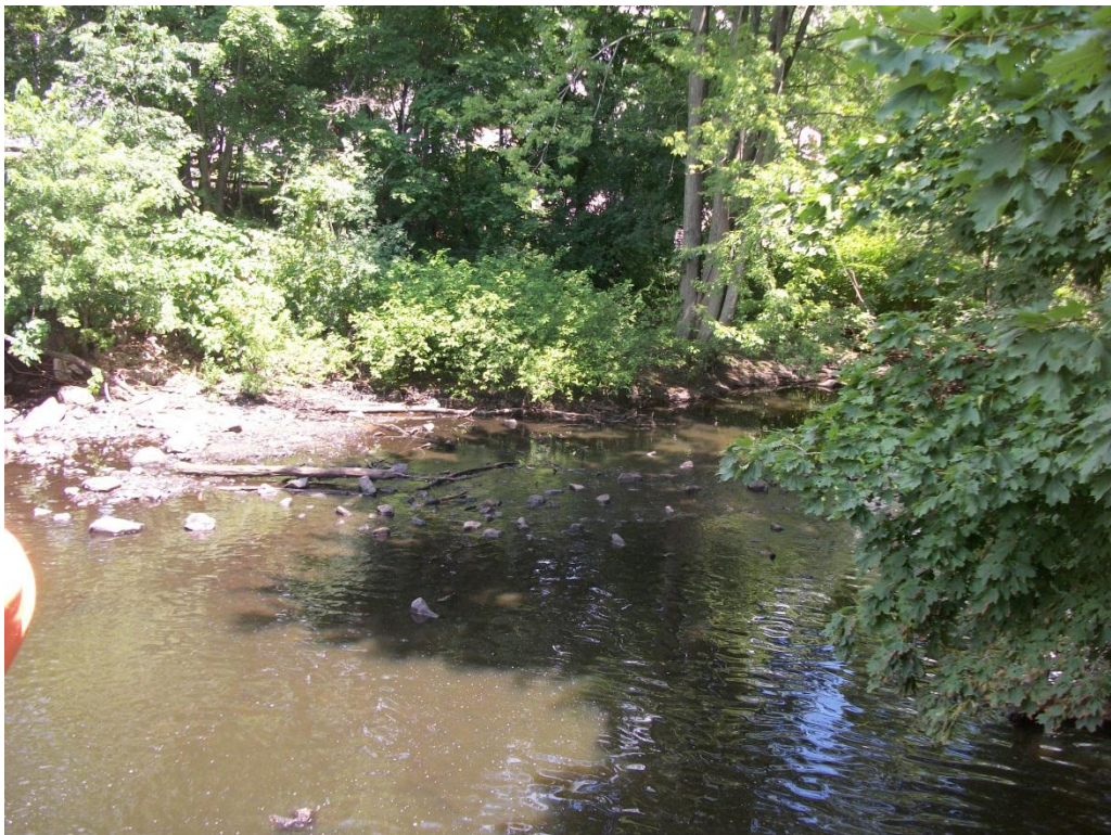
Photo 2: Downstream discharge channel from top of dam.
