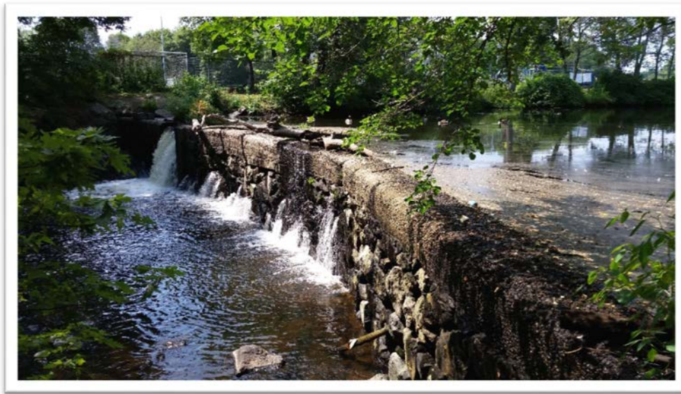
Colburn Street Dam (Looking South, Downstream)
