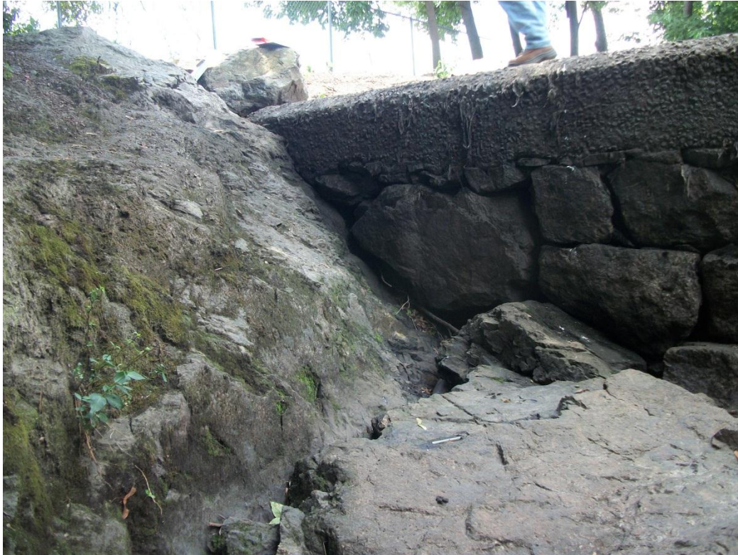
Photo 7: View of right abutment. Note good contact between concrete and bedrock.
