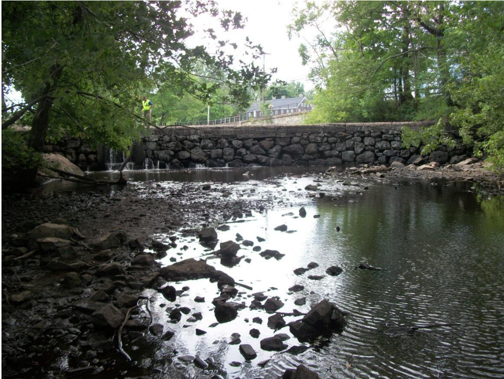
Photo 1: View of dam from downstream.
