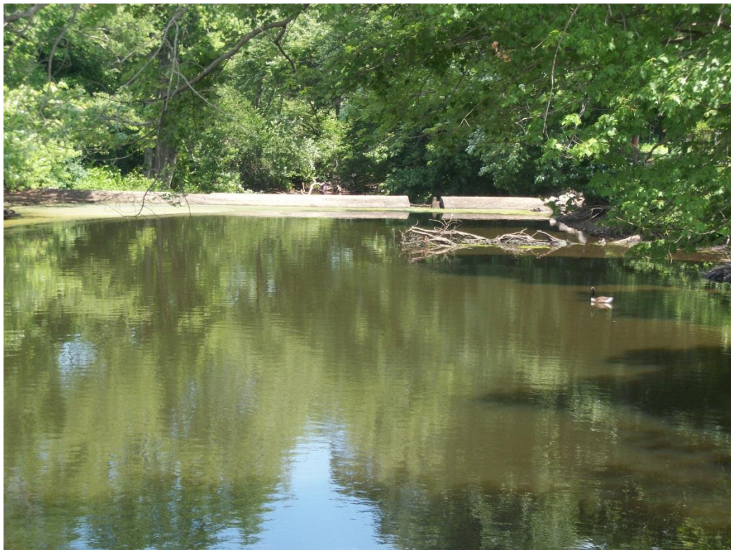
Photo 10: Upstream view of dam.
