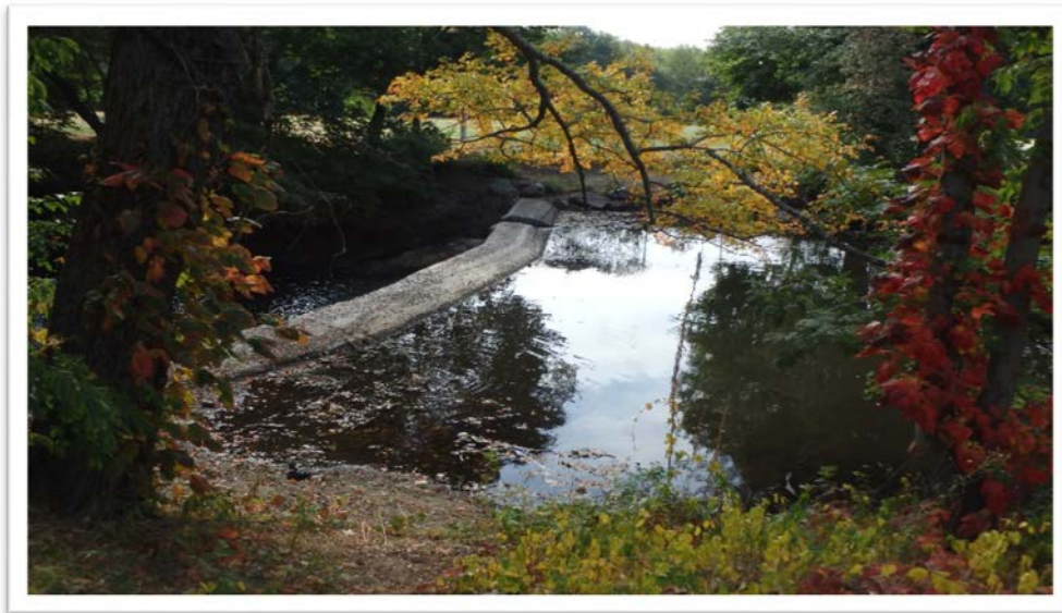
Colburn Street Dam (Looking South, Upstream)
